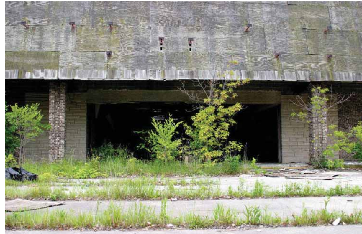
Dixie Square Hall, Harvey Illinois
