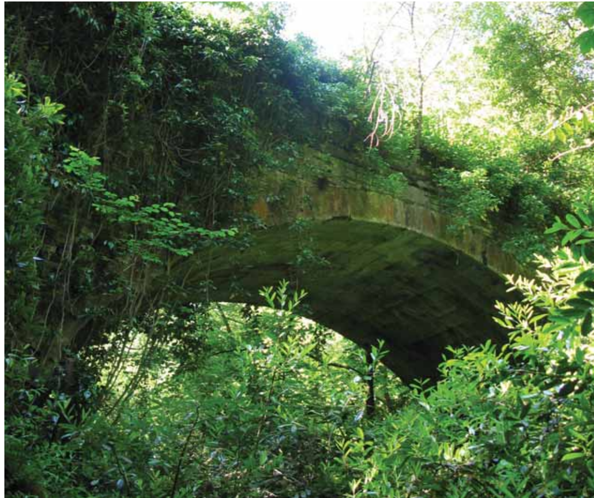
Kilmahew landscape - view from gorge up to main access bridge, photograph - James Johnson
